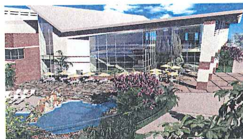
Highly-reflective roofing and hardscape materials limit the heat island effect. Image: Langdon Wilson.
